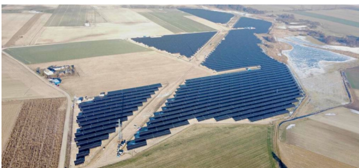
Raclawki, Solar PV
