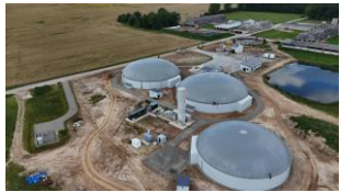
Launch of commercial biomethane production
