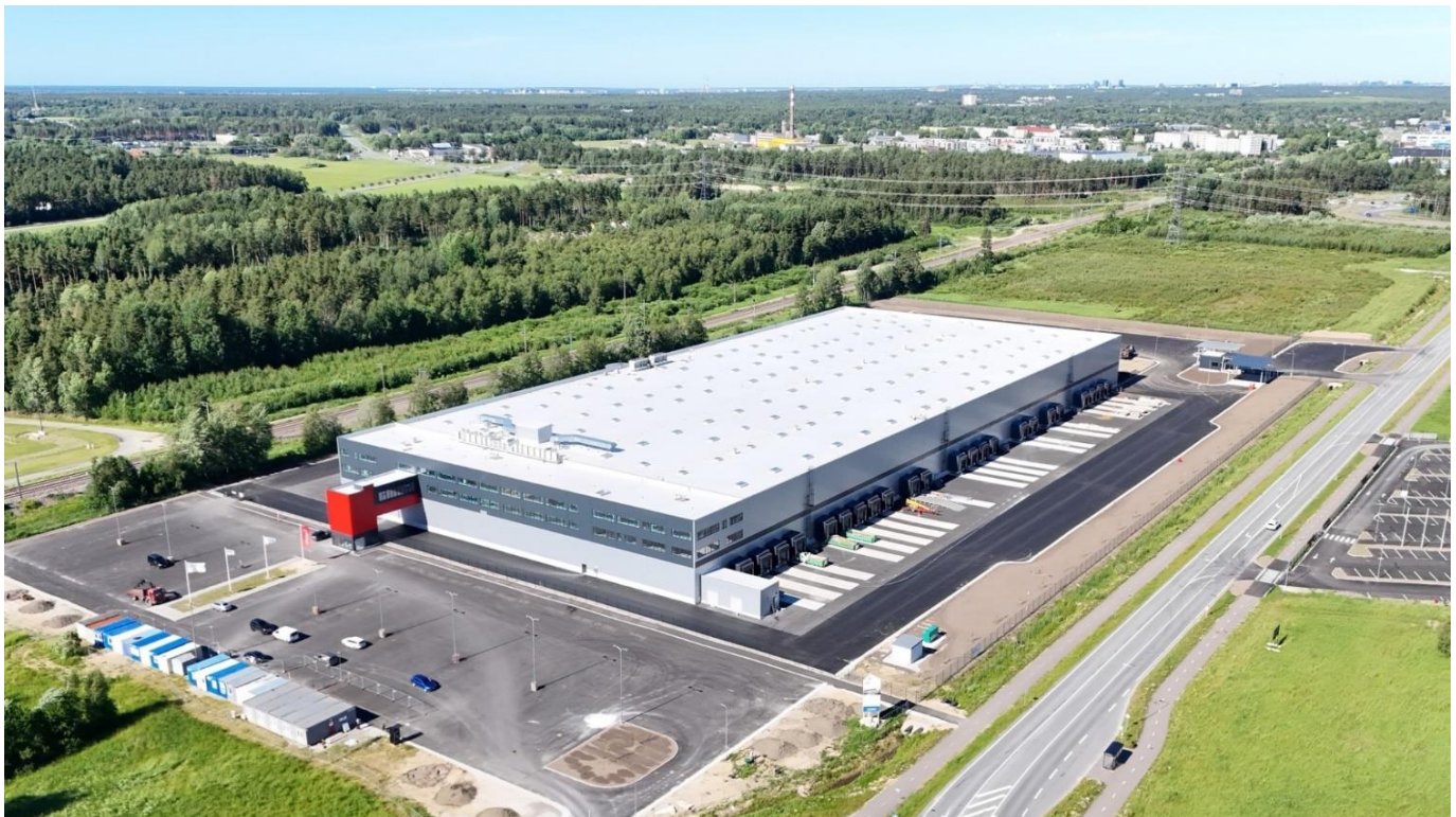
Construction of RIMI logistics centre in Saue, photo: Margus Kana
