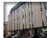
Office building in Vilniaus Street: GBA 9,800 m 2
