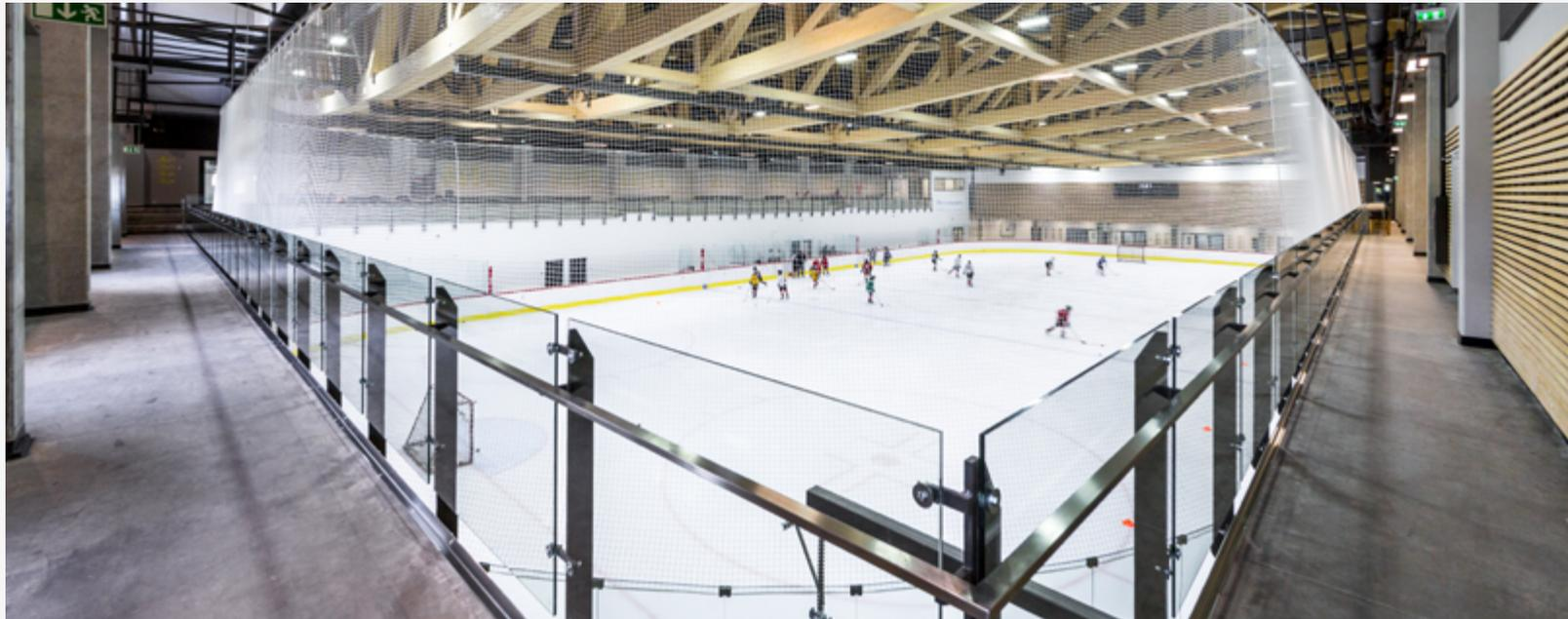
2014 COMPLETED MULTIFUNCTIONAL TONDIRABA ICE ARENA BUILT IN 14 MONTHS UNDER THE LEADERSHIP OF MERKO'S PROJECT MANAGER AHTO ARUVÄLI, WHICH INCLUDES THE MAIN ARENA, TWO TRAINING COURTS AND A CURLING ARENA. THE IMPRESSIVE WOODEN TRUSSES WITH UP TO 62 METER SPAN SHOWN ON THE PHOTO.
