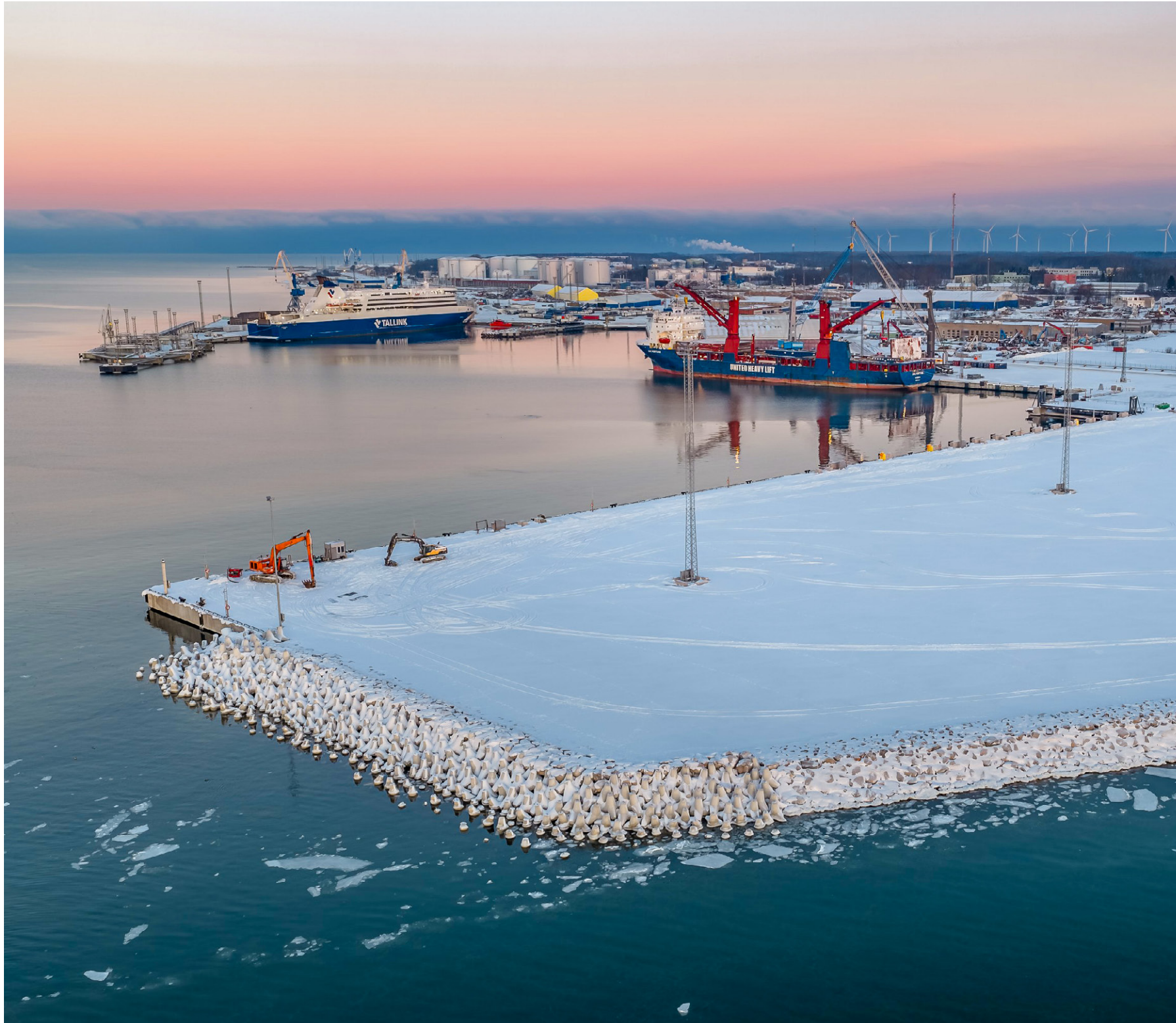
CONSTRUCTION OF THE NEW QUAY AT PALDISKI SOUTH HARBOUR WAS COMPLETED
